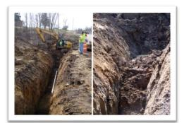
OSHA standards mandate that all excavations <u>5 feet or deeper</u> be protected against collapse. The employee was working in a trench at a depth greater than 10 feet without cave-in protection. OSHA's investigation is ongoing. The agency will determine why the job was being done in this fashion and what, if any, violations occurred.
